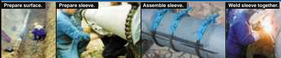
Pipe is cleaned. Epoxy is applied. Sleeve is assembled, brought to the required compression, and welded together ... all in about an hour.
